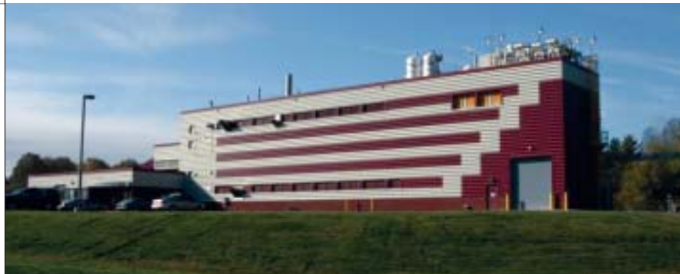
The National Corn-to-Ethanol Research Center, located at University Park, a research park on the campus of Southern Illinois University Edwardsville, is the only facility in the world that fully emulates both a corn wet-mill and dry-mill commercial ethanol production center. Sixteen trials are currently underway.
